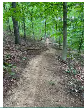
SCA Trail Build
